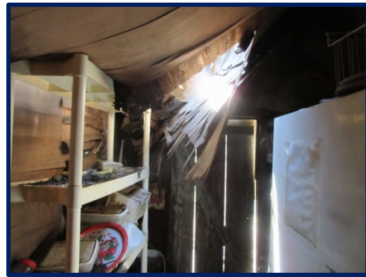
Interior View of Storage Building
