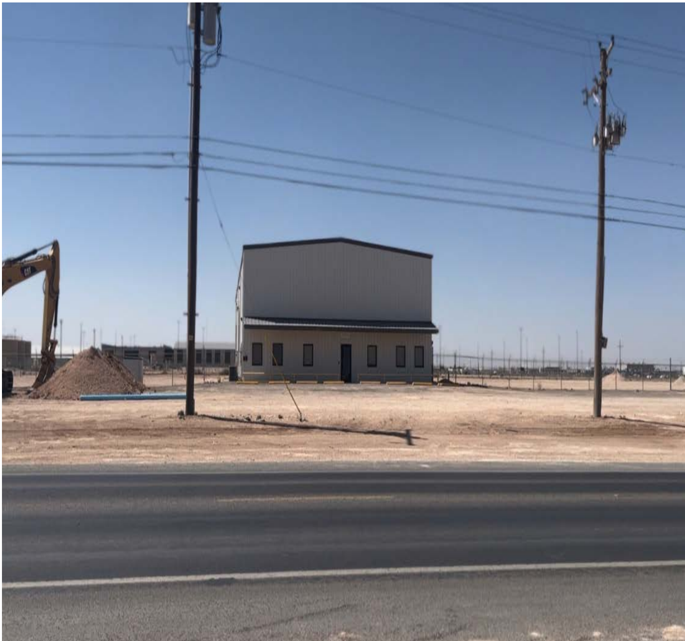
On Farm to-Market Road 715, Looking West
