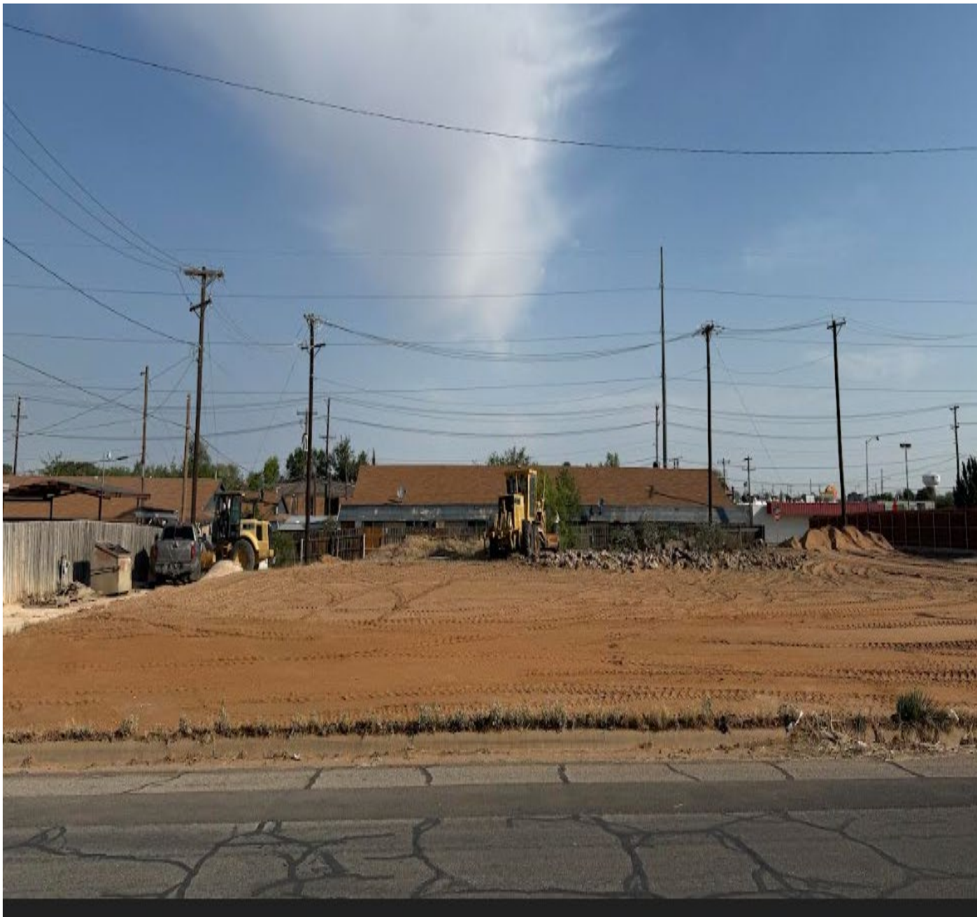
On George Avenue, Looking North
