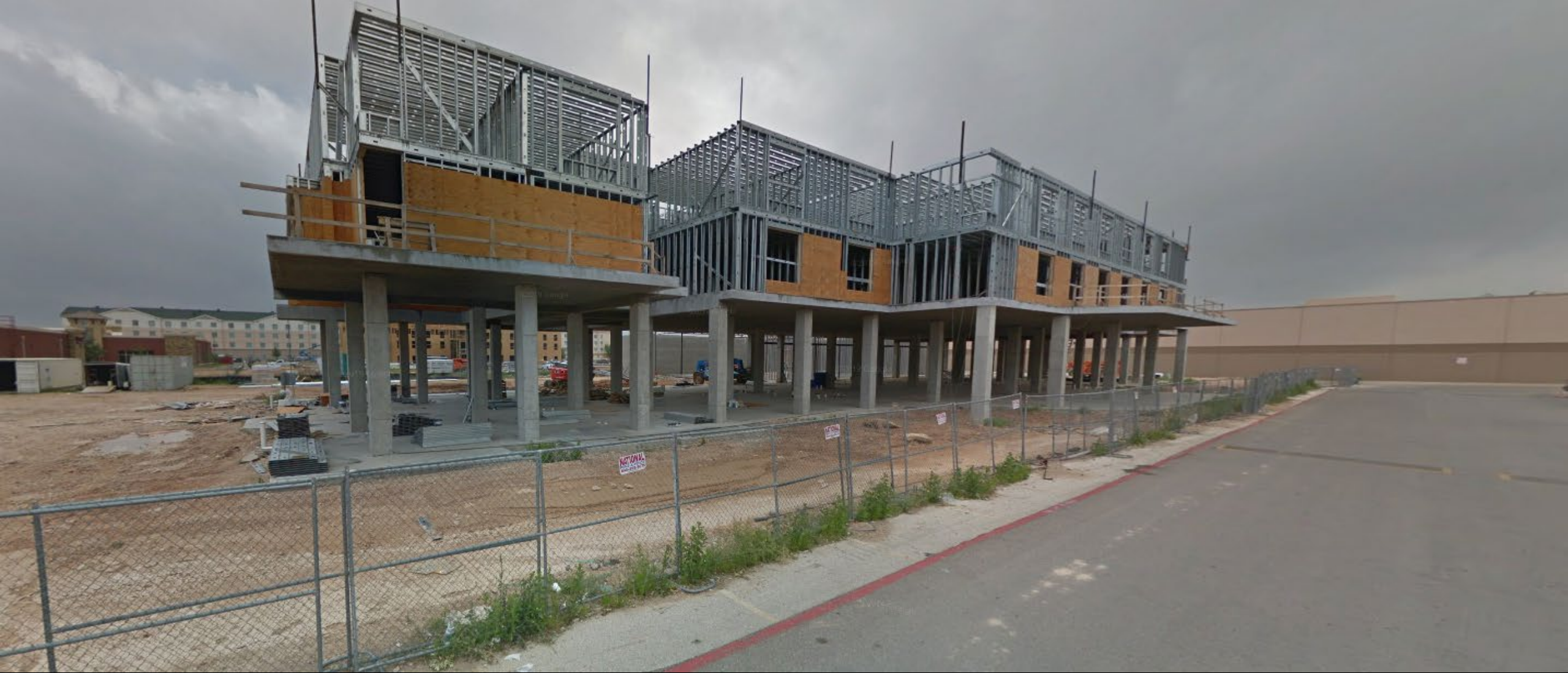
On HEB (Parking Lot), Looking Northwest
