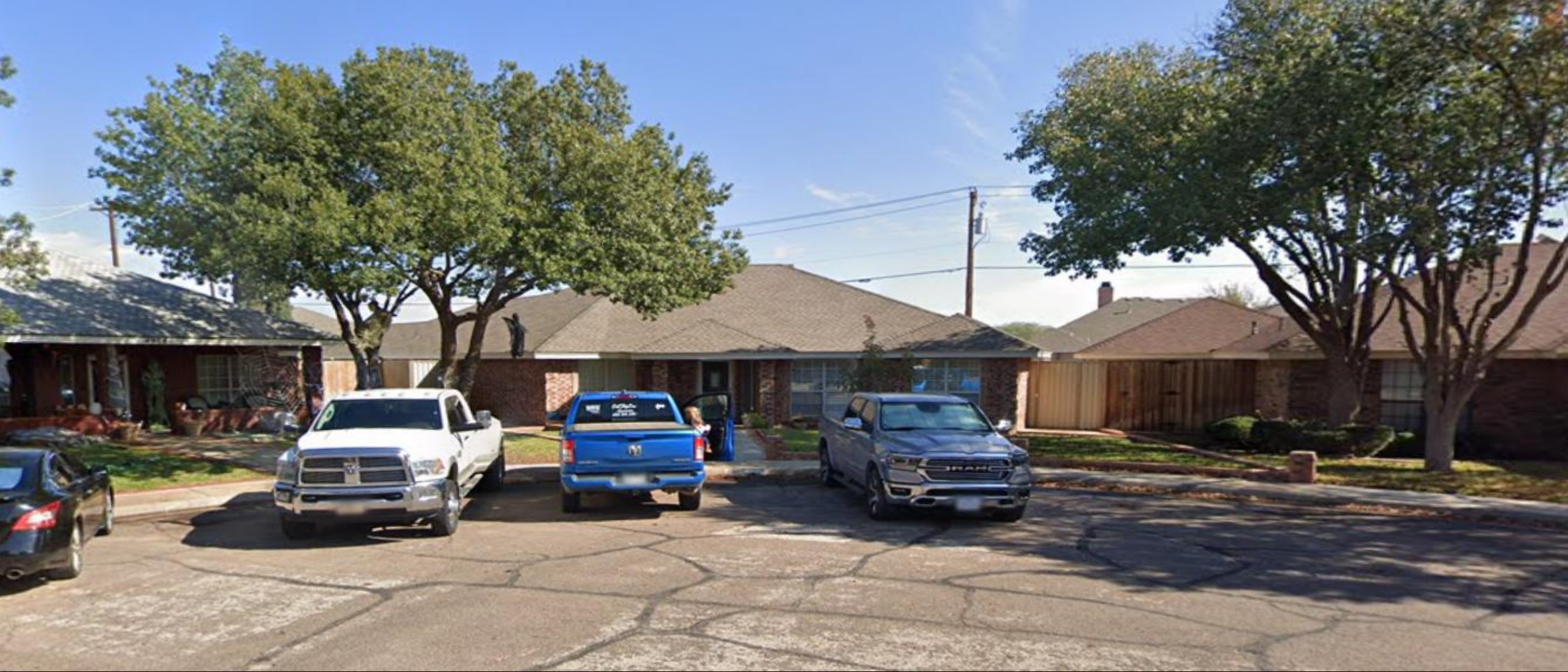
On Timber Court, Looking East
