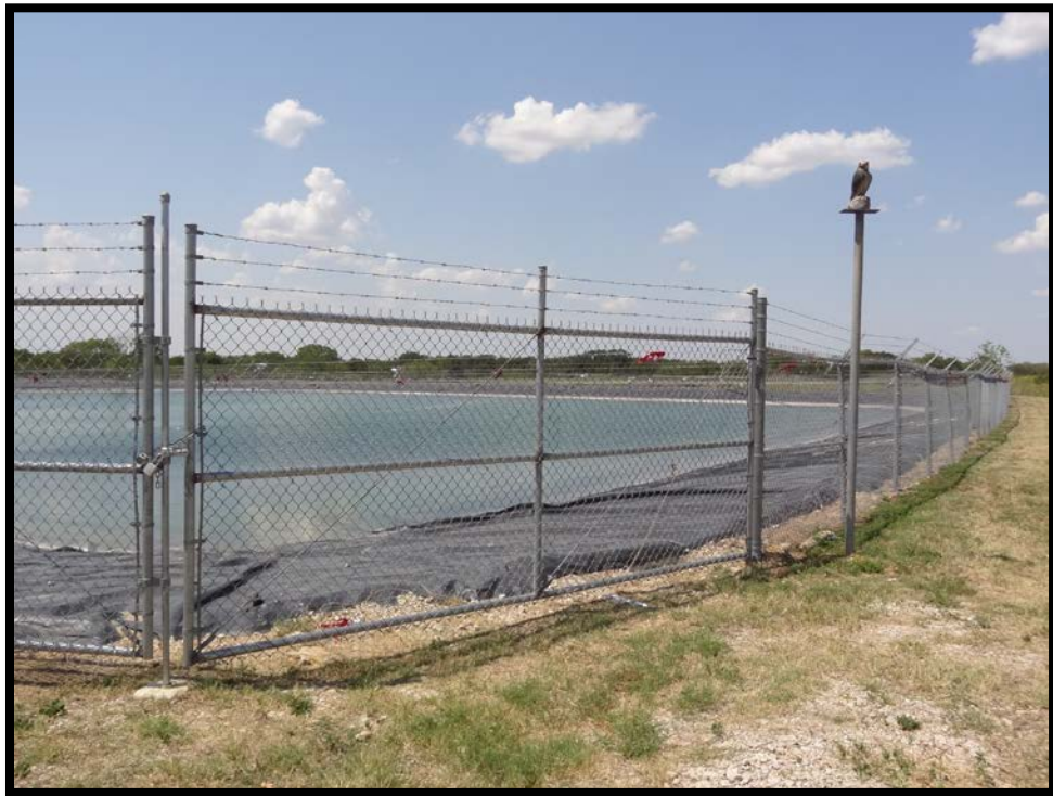
Photo 6. At DFW, the wire grid is attached to the chain-linked fence to prevent birds from walking beneath the wires. Credit: Marcelino Sanchez/FAA
