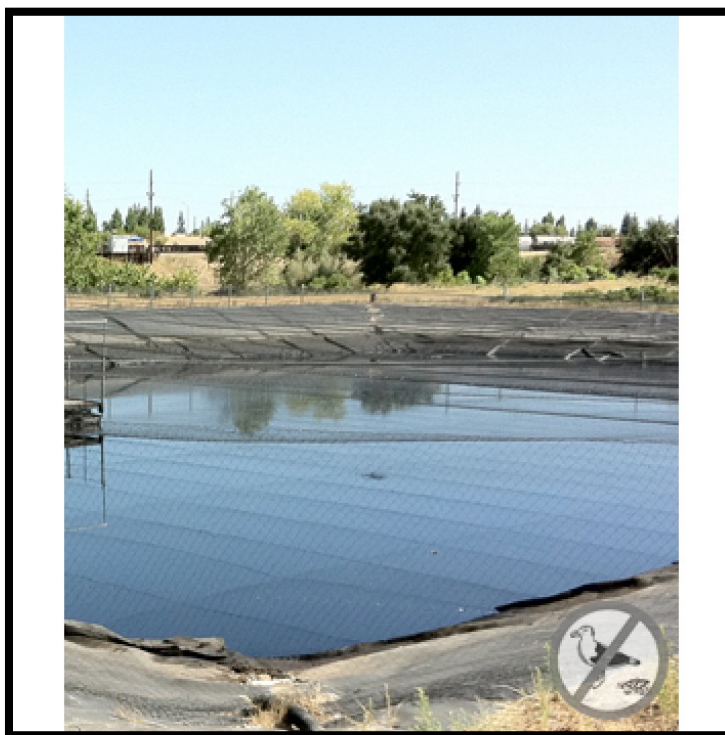
Photo 8. Representative photograph of industrial netting across a retention pond. Credit: www.Birdbgone.com
