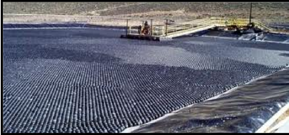
Photo 7. Representative photograph of Bird Balls™ placed in a retention pond. Credit: www.paradisew.com
