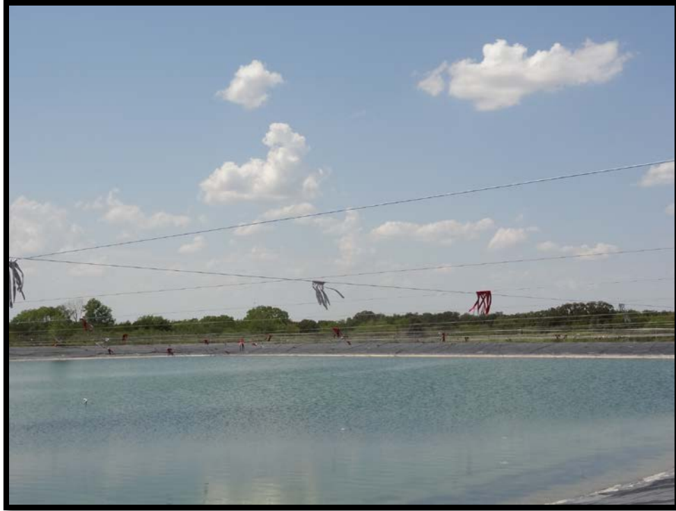
Photo 5. Wire grid with streamers placed above a retention pond at Dallas-Fort Worth Airport (DFW). Credit: Marcelino Sanchez/Federal Aviation Administration (FAA)
