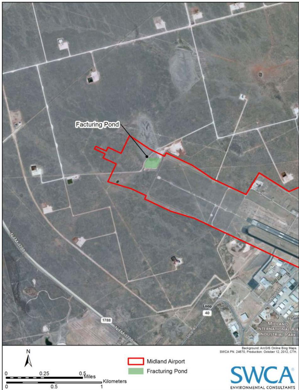
Figure 2. Aerial view of the fracturing pond at Midland International Airport.
