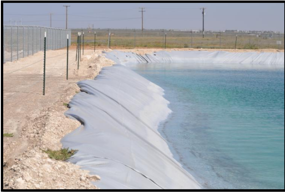
Photo 3. The steep banks of the fracturing pond with the three-strand barbed-wire fence surrounded by the 6-foot chain-link fence. Credit: Olivia Münzer/SWCA
