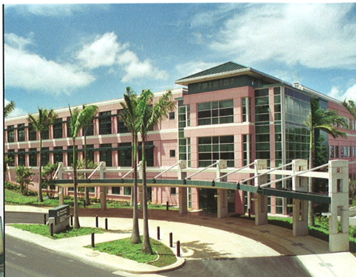
VA Medical Regional Office, Honolulu, HI - Architects Hawaii, LTD.
