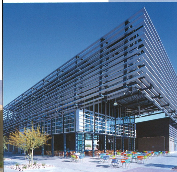
Chandler Gilbert CC Student Center, Gilbert, AZ - Architekton
