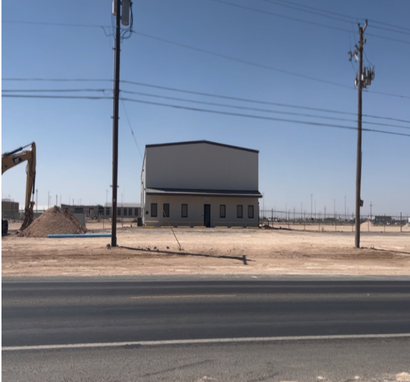
On Farm to-Market Road 715, Looking West
