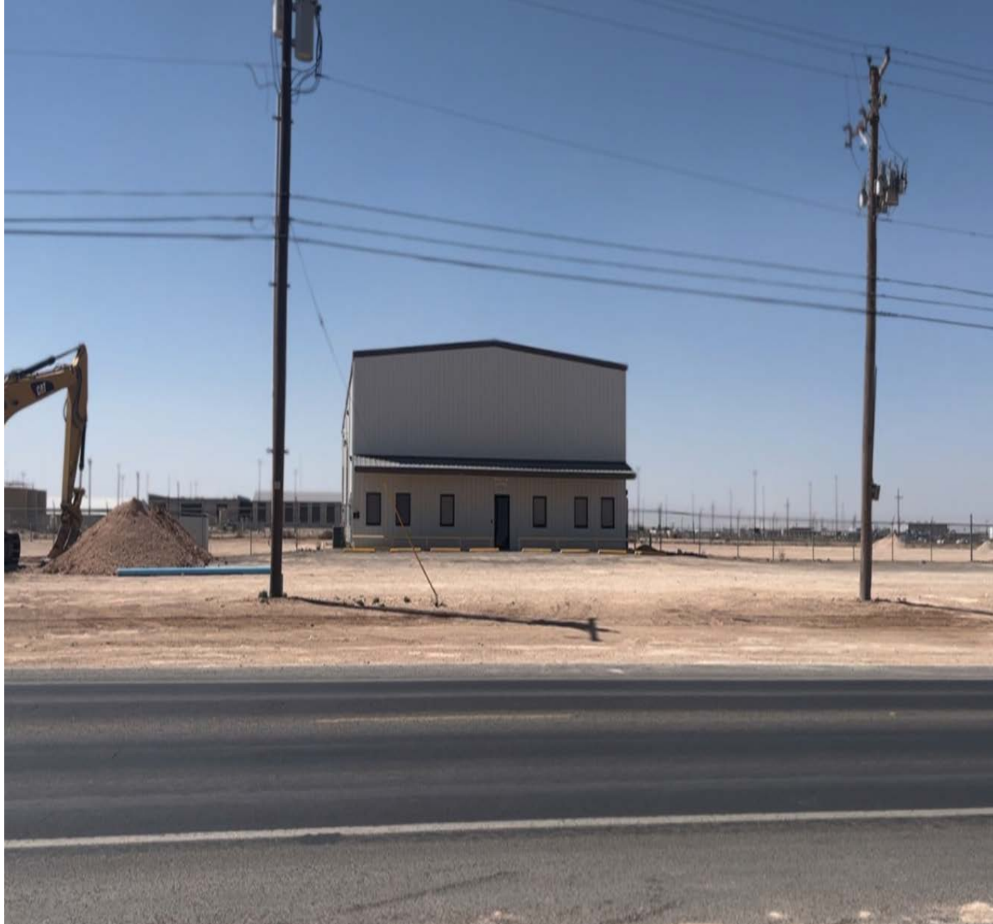
On Farm to-Market Road 715, Looking West
