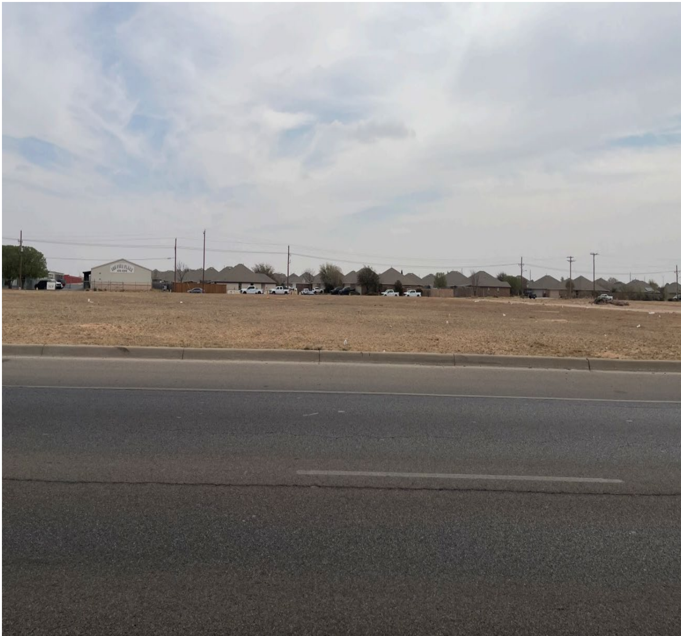
On North Big Spring Street, Looking East
