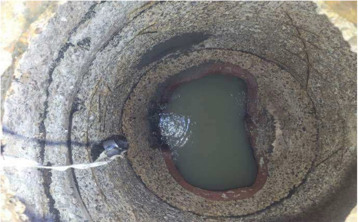
EXIST CONCRETE MH PRESSURE WASHED
