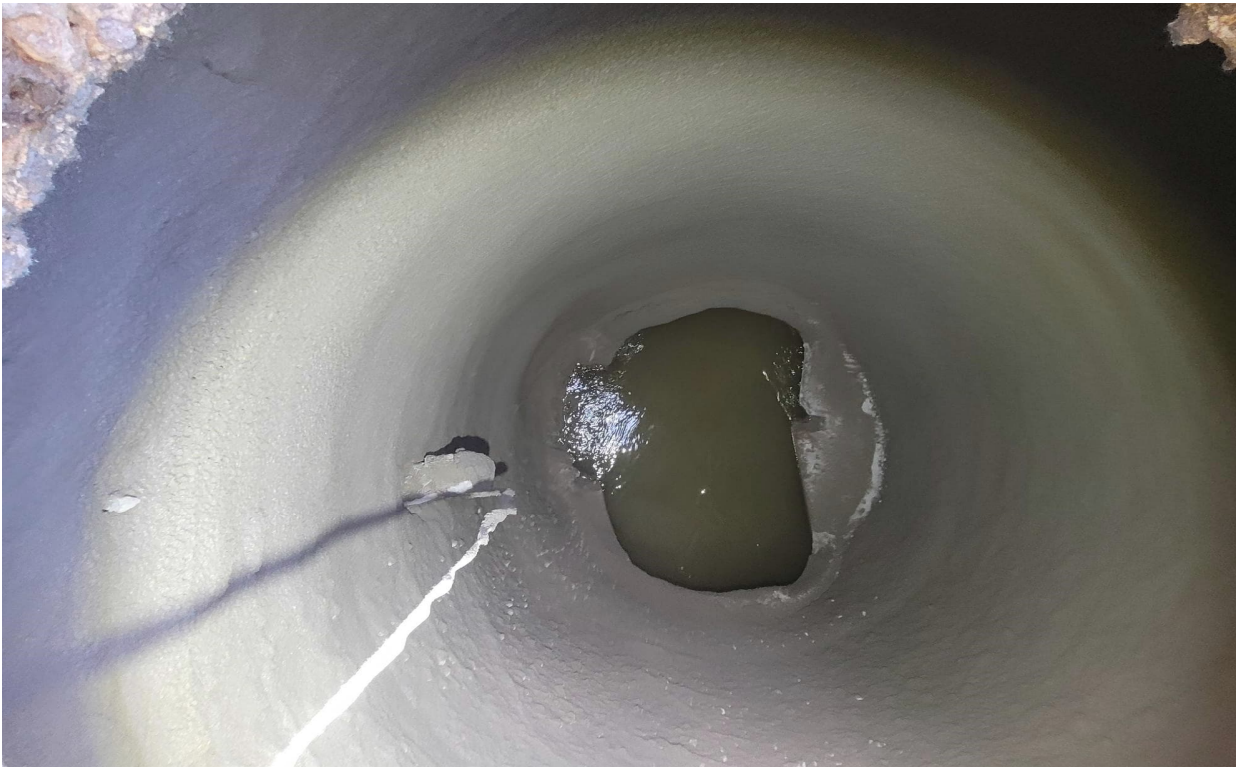
CONCRETE MH REHAB INVERT SHAPED & INVERT/MH LINED
